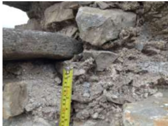
Views of mortar in the wall core areas
