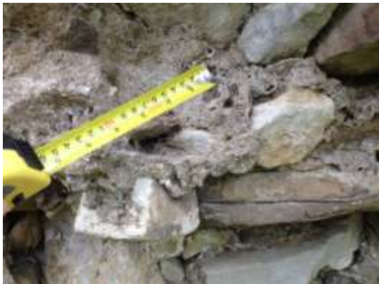
Views of mortar in the wall core areas
